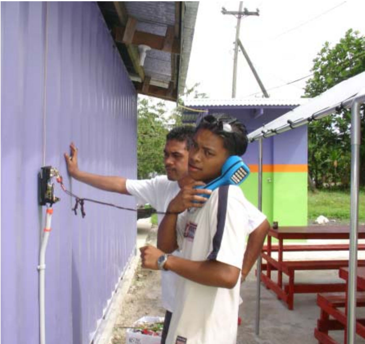
Telecommunications students at College of Micronesia-FSM, Pohnpei Campus testing a new telephone line.
