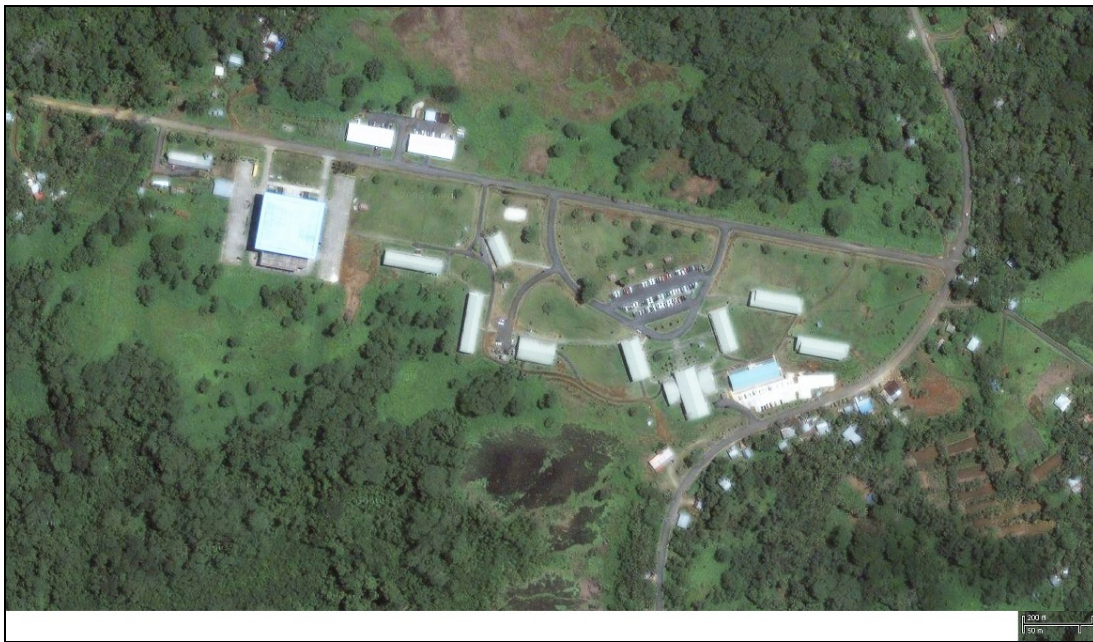
Figure 2. Aerial view of COM-FSM National Campus. 2013. Photo courtesy of Beca. Note that the overall footprint of even the National Campus is compact and should make face-to-face communication relatively easy.
