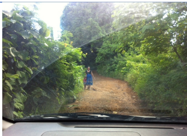
Access on a slope on leaving Pou to reach the Nantaku site – single lane unsealed road, susceptible to rutting due to lack of drainage
