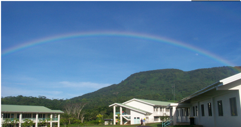
Side view of classroom buildings and newly constructed faculty building
