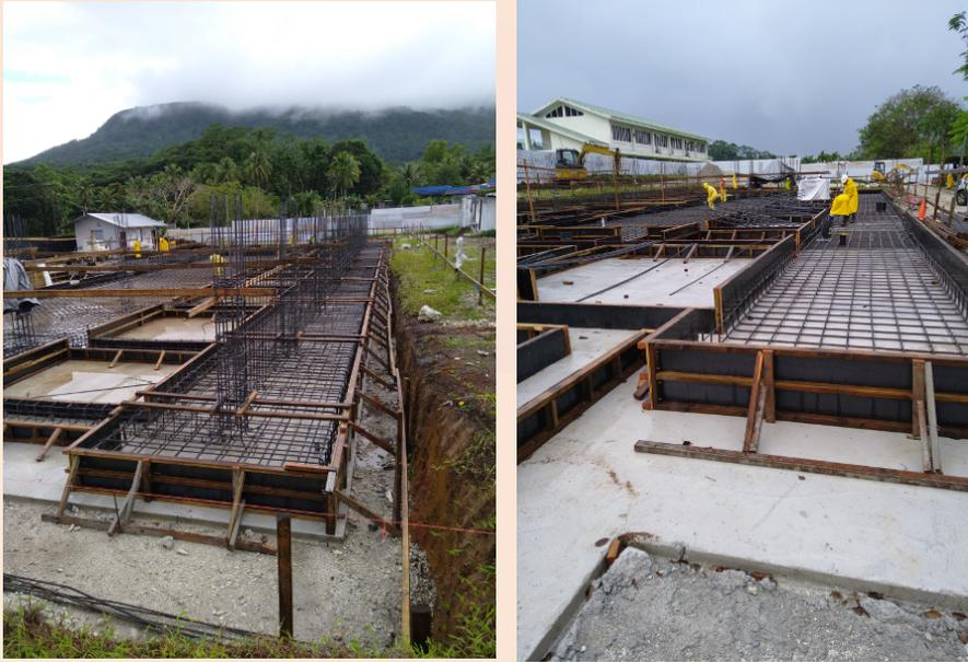
**National Campus Student Center:** Building Concrete base is complete and waiting for reinforcement bars for the foundation works to arrive. Meanwhile the contractor is constructing concrete masonry blocks. Refer to images below
