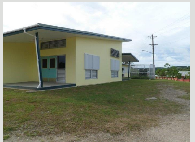
Use existing roof areas on new buildings for addition solar power
