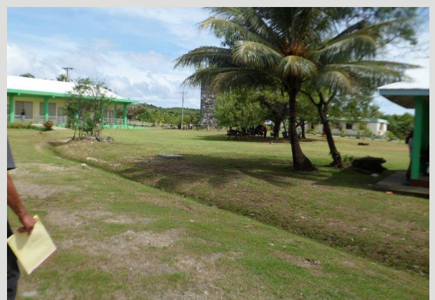
Drainage channel through the Center of the campus - landscape treatment and pedestrian access across needs to be considered
