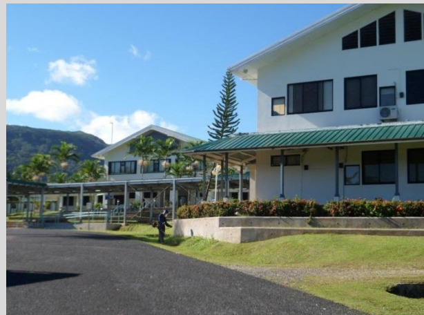
The planting of the palms in front of the LRC building show how the use of indigenous planting can be successfully implemented on the campuses
