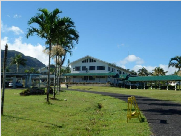
Swales alongside the entry road – bridging across at points make students access the front lawn area more
