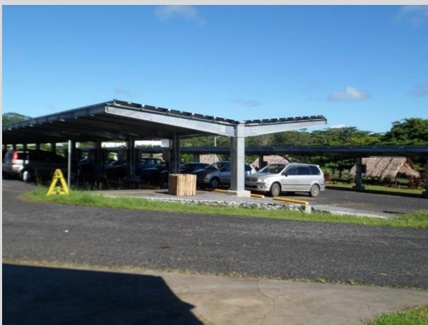
Front main car park with solar panel structure providing dual function of shade and power generation
