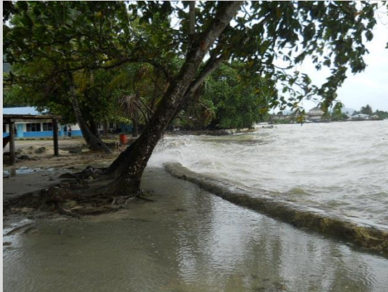
Exposure of the current site to storm surges with flooding of the buildings close to the sea frontage
