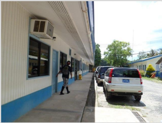
Eaves form cover over length of the main buildings
