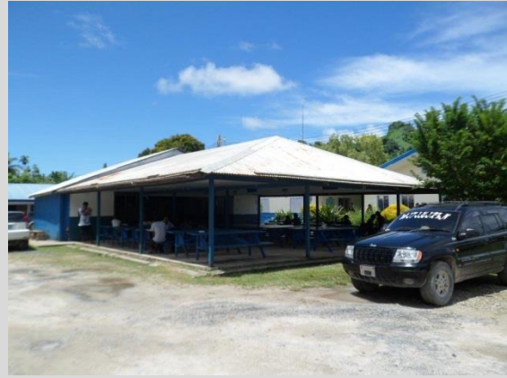
The student center is the focal point of the campus
